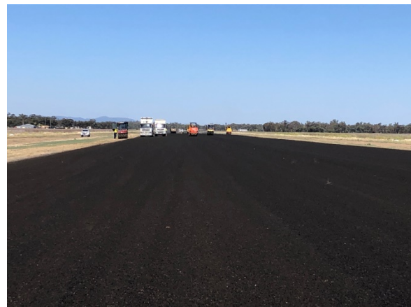
Airport Tarmac Upgrade underway
