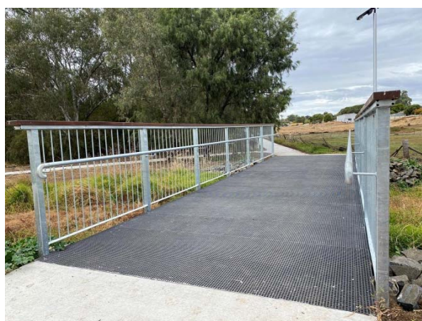
Stormwater bridge along the new Riverine Stormwater Precinct Shared Pathway project.
