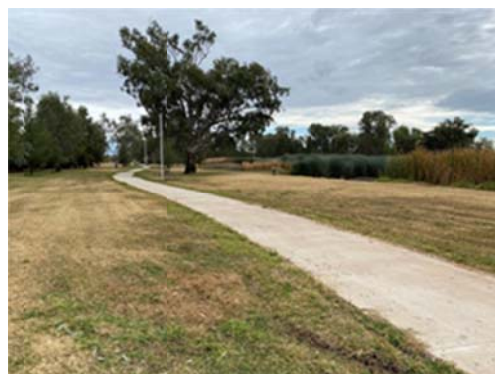
Riverine Stormwater Precinct Shared Pathway.
