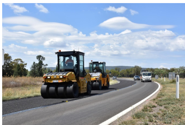
Roadworks being completed on Kamilaroi Highway near Curlewis.
