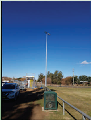
Light poles installed at Donnelly Fields
