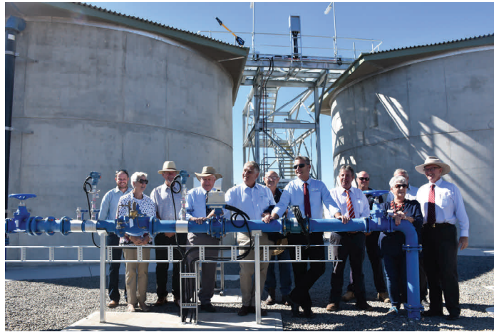
Official opening of the Curlewis Pipeline
