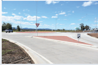
Boundary Road Roundabout completed by Council staff.
