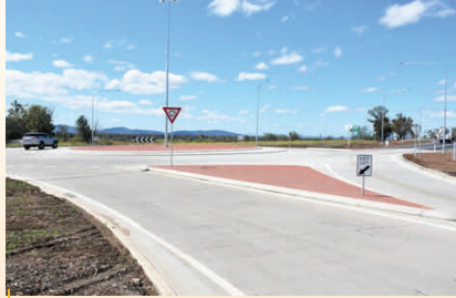
Boundary Road Roundabout on the Oxley Highway
