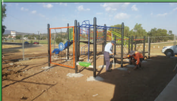
Installation of playground equipment at Donnelly Fields
