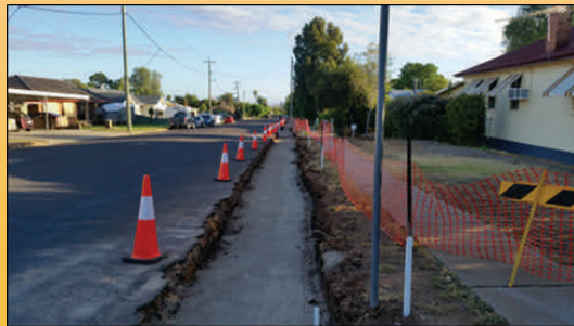
Bridge Street kerb and gutter construction works
