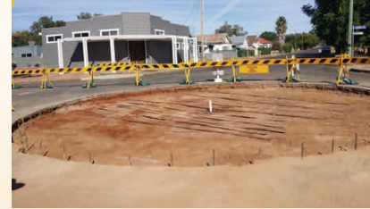
Boundary Road Roundabout on the Oxley Highway
