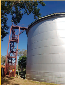
Works being completed on the South Street Reservoir
