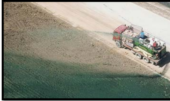
Figure 3 – Hydromulch application (Spraygrass 2009)
