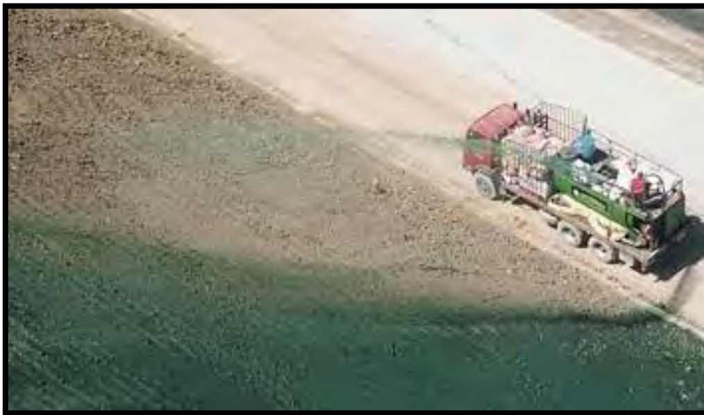
Figure 2 – Hydromulch application (Spraygrass 2009)
