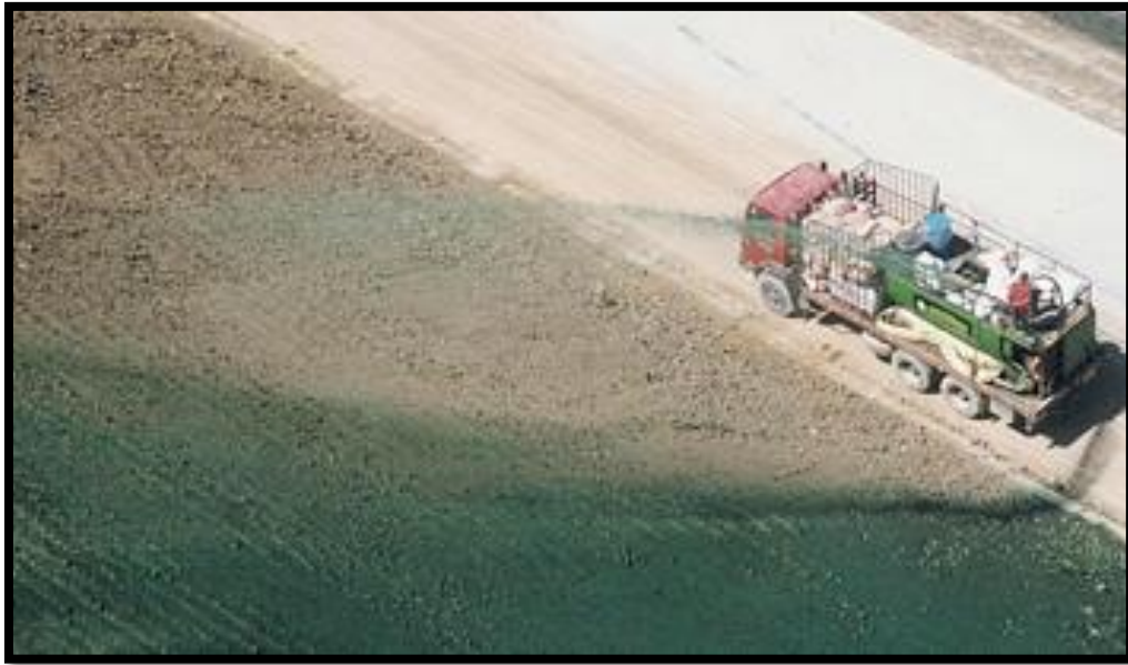
Figure 3 – Hydromulch application (Spraygrass 2009)
