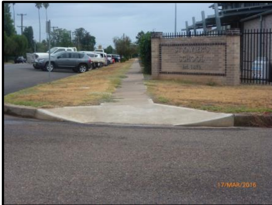
Plate 8 - Typical kerb ramp
