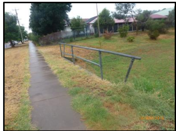
Plate 7 - Typical Concrete Footpath
