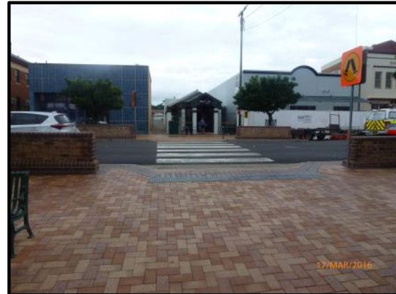
Plate 9 - Kerb ramp with tactile marker
